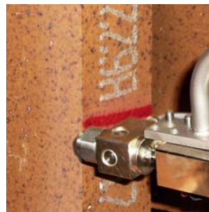
Chimney stone line-marking for correct installation
